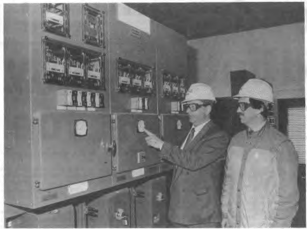
Contracting 1st Engineer Colin Arnold (left) and Network Services 2nd Engineer Tony Hassall (both based at Mid-Mersey) checking equipment in the BA Alloys substation.
